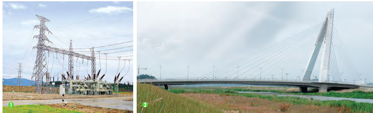
1 Young-Am S.S. construction project 2 Nam-Chang Grand bridge, Stand-by power cable installation
